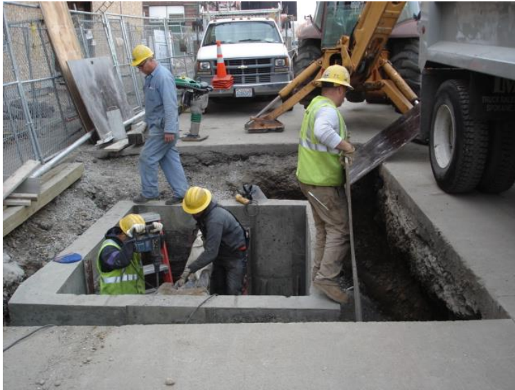
Figure 27, Complete replacement of a badly deteriorated manhole
